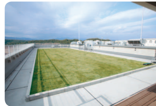
Grass is grown in two places on the roof of the factory, which is watered with rainwater.
